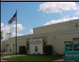
Filtration Plant on North Lake Street
