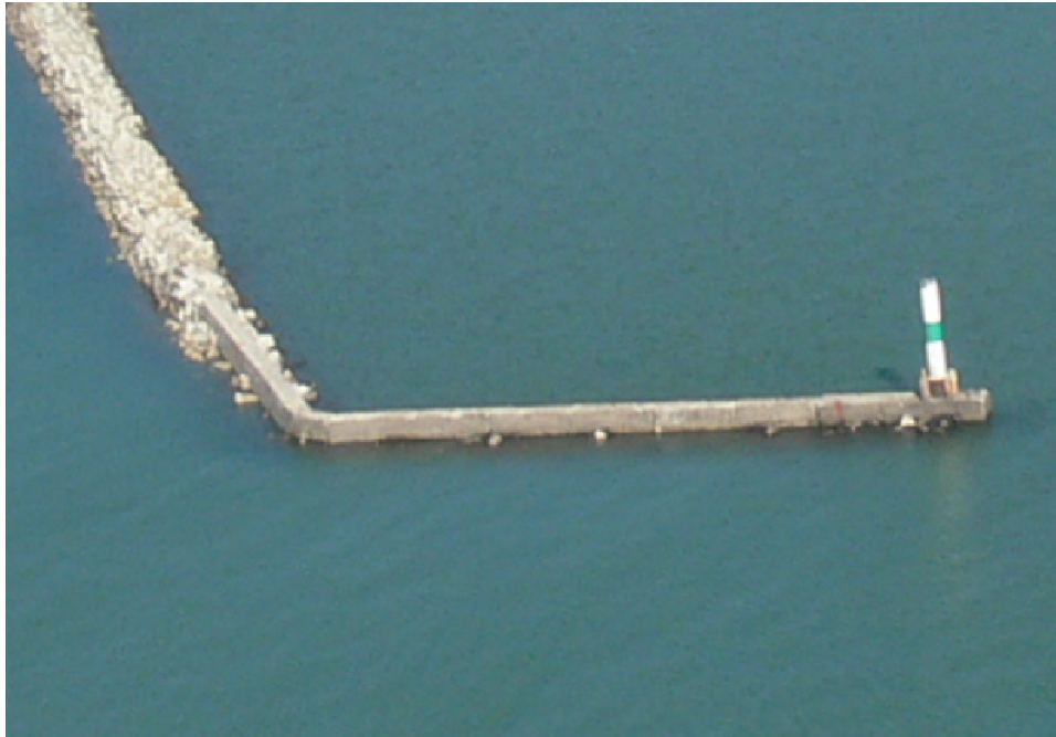
Aerial photo of the South Breakwater, sections J and A (federally-owned)
