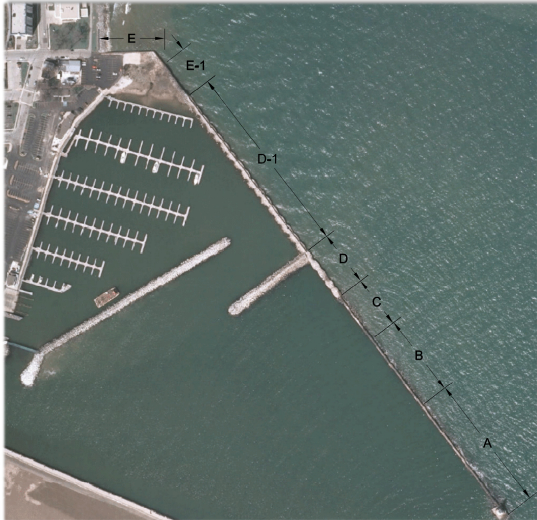
Aerial photo of the North Breakwater, sections E through A
